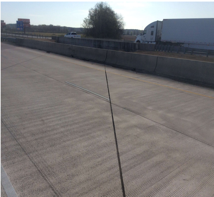
PHOTO 1 Description Bent #2,3 poured joint seal has a few spots of loss of adhesion ten feet total.
